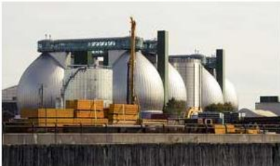
Industrial scale egg shaped digesters near NYC, USA used for waste water treatment.
